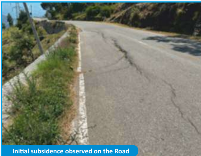
Prominent Cracks developed on the pavement
