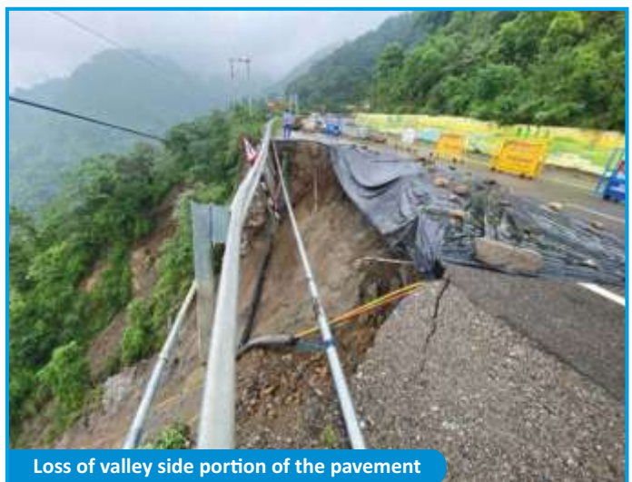
Prominent Cracks developed on the pavement
