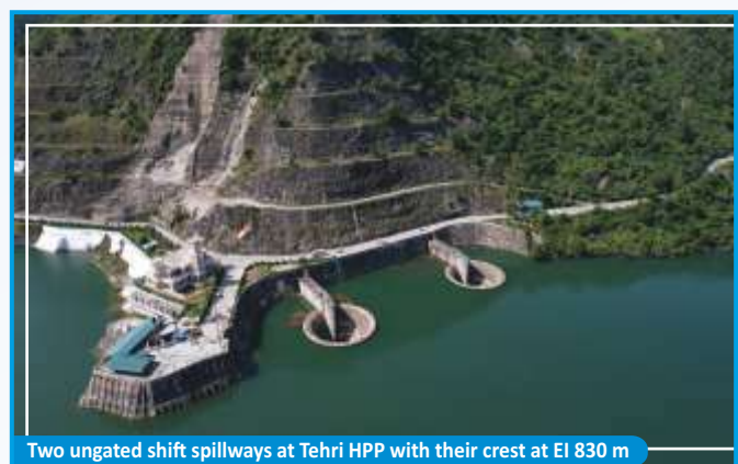
Two ungated shift spillways at Tehri HPP with their crest at El 830 m
