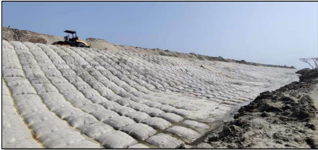
Fig.-2-Image showing installed Articulating Grouted Concrete Mattress over canal slope protection
