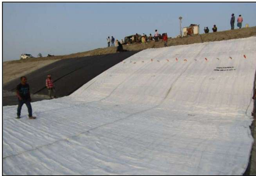
Fig.-5-Laying of fabric
