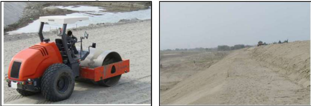
Fig.-3-Preparation of subgrade before installation
