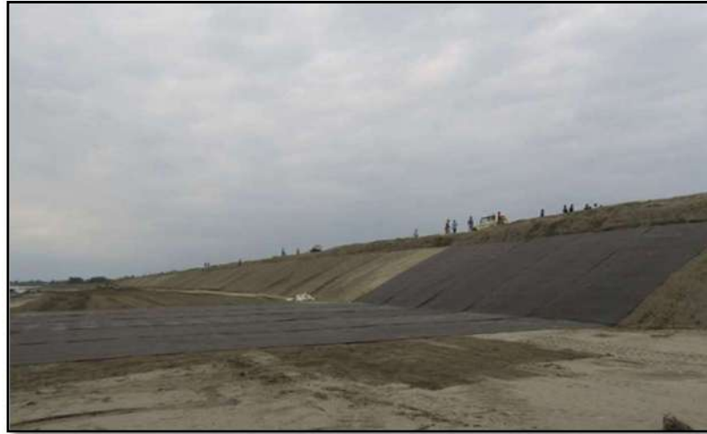
Fig.-4-Laying of Geotextile layer
