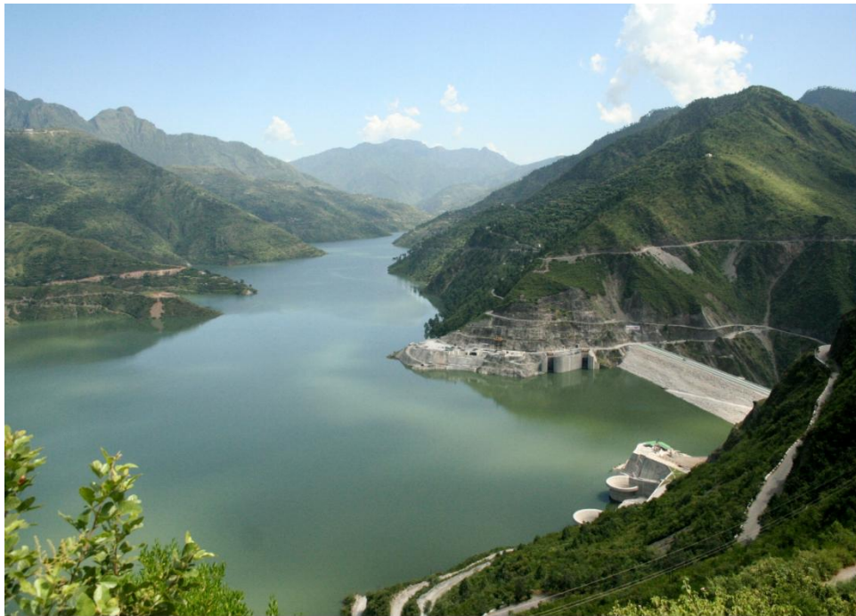
Fig 2 View of Tehri dam and its Chute Spillway
